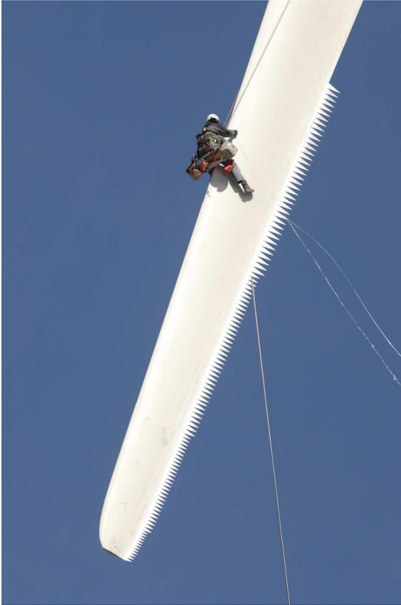
Figure 1. Climber removing trips from serrated blade.
